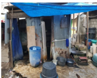
Insufficient community toilets and septic tanks
