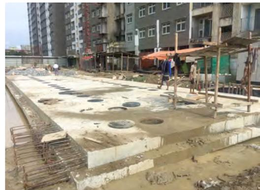
■ Installation of manholes and selection of filter stoned for DEWATS unit 2
