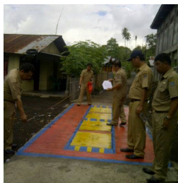
Community-based DEWATS plant
