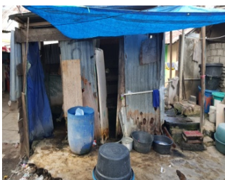
Insufficient community toilets and septic tanks
