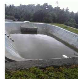
Sludge Treatment Plant
