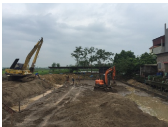
Starting the construction of wastewater treatment plant
