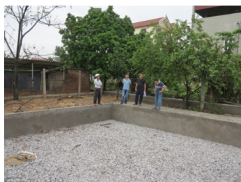
BORDA – VAWR engineers supervised the construction
